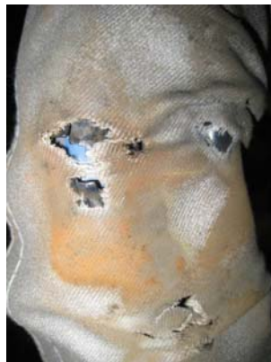
Fig. 1.2.2 (b) Damages on the cable protective sleeve
